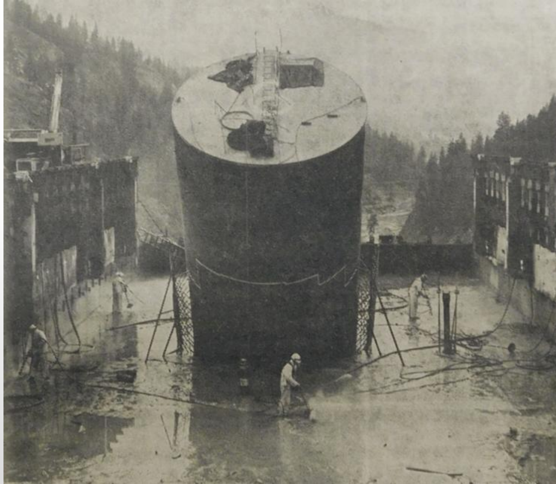
Dworshak Dam construction, penstock tube, Clearwater Tribune, February 5, 1970
